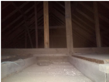
Ceiling supported by raised tie trusses
